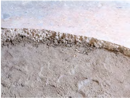
Fig. 18.3 Lhasa, Jokhang. Clay (in front) as sub-layer.
