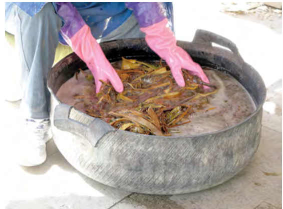
Fig. 35.3 Lhasa. Gyüme Dratsang. A sirup-like doughly liquid remains for impregnating the roof.
