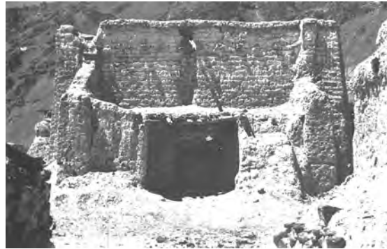
Fig. 6.2 Tabo. South elevation of the Maitreya Lhakhang. Source: Khosla (1979: plate 44).
