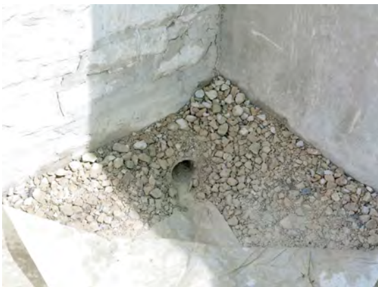
Fig. 28.3 Lhasa. Gyüme Dratsang. Corners and sprouts are rammed and smoothed last.
