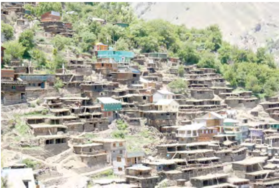
Fig. 1.3 Labrang, Kinnaur, India. Flat roof constructions.
