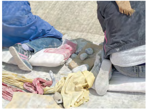
Fig. 27.3 Lhasa. Gyüme Dratsang. For smoothing each worker has own preferences in size and form of the polishing stone.
