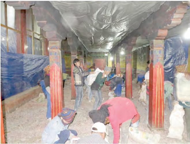
Fig. 36.3 Lhasa. Gyüme Dratsang. Renewing the old concrete floor with arga .
