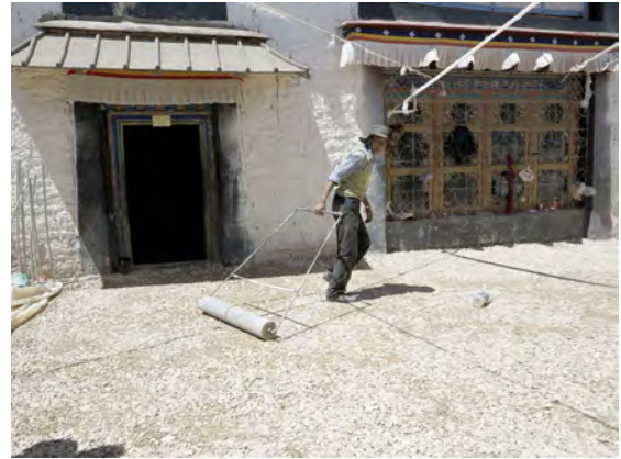
Fig. 19.3 Gyüme Dratsang. Stone roller for compression.
