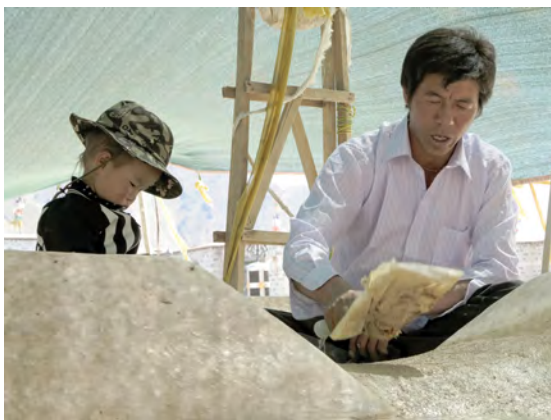
Fig. 22.3 Lhasa. Gyüme Dratsang. Preparing the attic with a lakchak .
