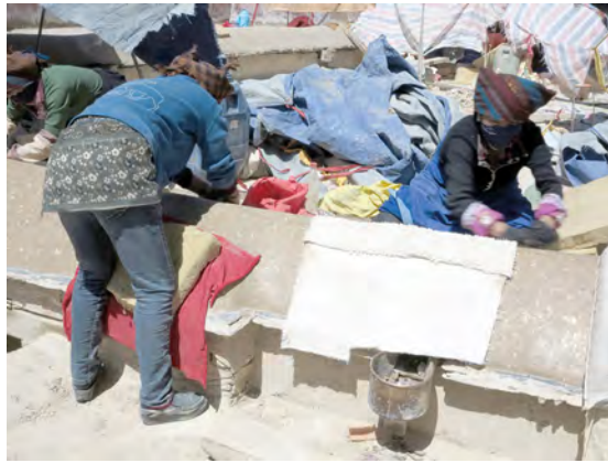
Fig. 31.3 Lhasa. Gyüme Dratsang. Protecting the moistened attics against the sun.
