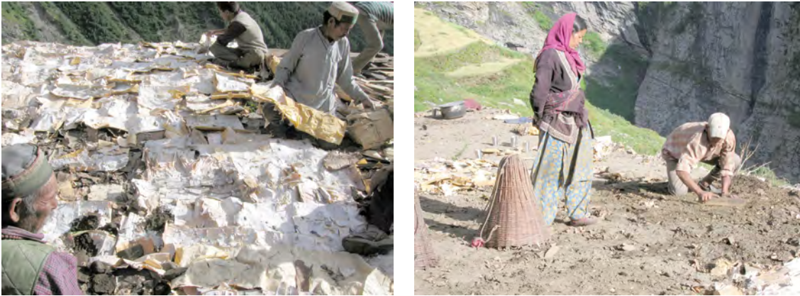
Fig. 9.3 (Left) Purthi. Chamba. India. Birch bark as organic layer below the clay.
