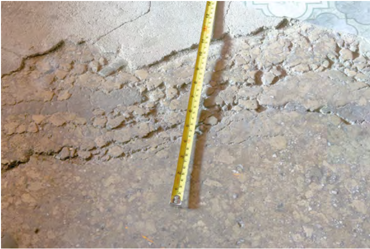
Fig. 5.3 Spituk. Ladakh. Assembly hall. Arga partially covered with PVC.
