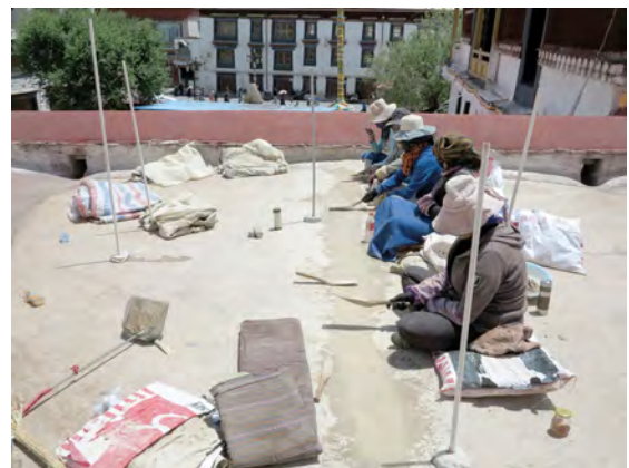
Fig. 23.3 Lhasa. Jokhang. Stitching cracks in the arga roof with a lakchak .
