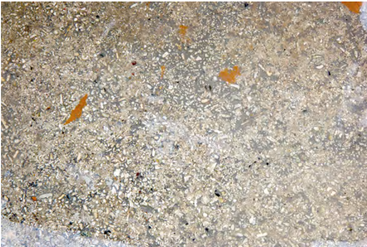
Fig. 6.3 Lamayuru. Ladakh. Zimchung . Arga after removing the covering PVC floor.
