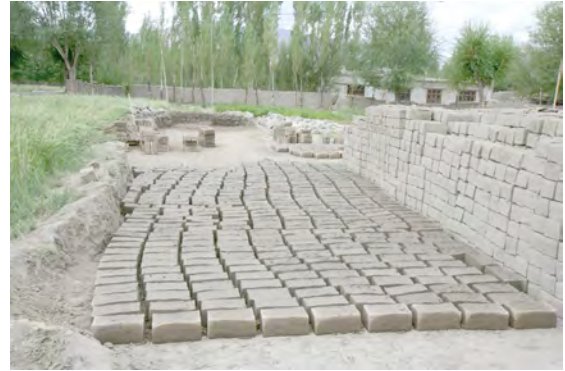
Fig. 4.2 Nyarma. Bricks laid for drying.
