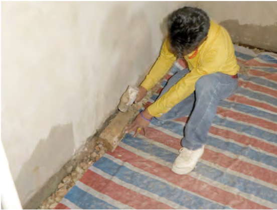
Fig. 24.3 Lhasa. Gyüme Dratsang. Preparing corners separately with wood block and hammer.
