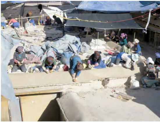
Fig. 26.3 Lhasa. Gyüme Dratsang. Smoothing the attics by burnishing with stones.
