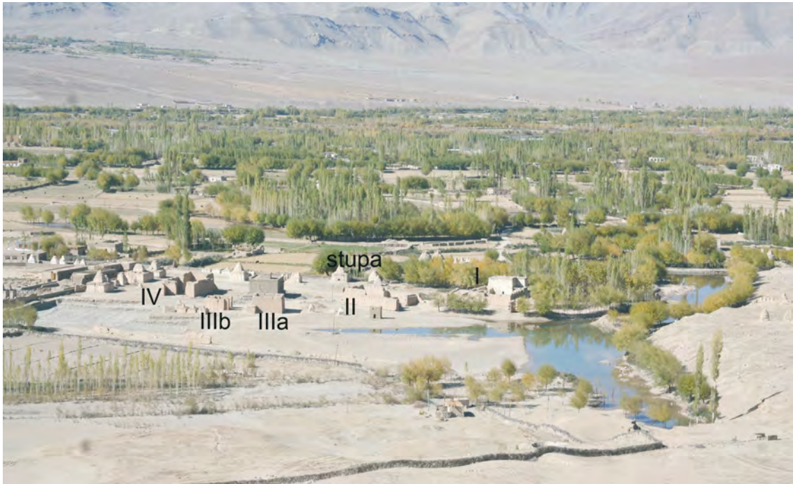
Fig. 2.2 Nyarma Monastery. East view. Numbers of structures according to the groundplan in Fig. 1.2. Source: Feiglstorfer (2011: Abb.4). I = main temple including attached structures V, VIa and VIb (which are not marked on the picture). II, IIIa, IIIb and IV = temple structures. Stupa = accessible stupa within the monastery compound.
