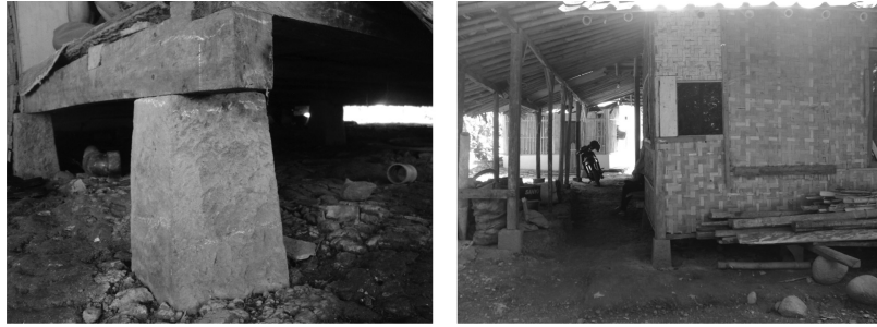
Figure 3. Stilt house. (Source: personal documentation).
