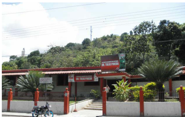
Figure 10. Community Hospital in Guárico state where the Comprehensive Medicine Study Program is offered (Source: own photograph in 2012)
