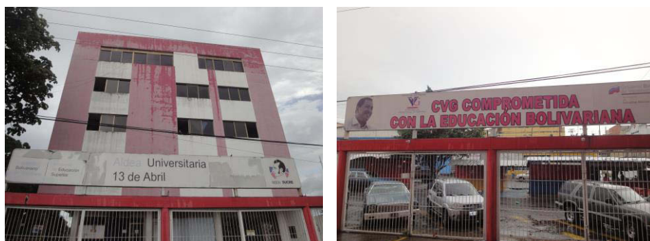
Figure 11. Multipurpose building where different Missions coexist in Bolívar (Source: own photographs in 2012)
