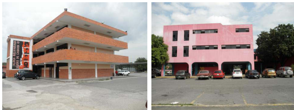
Figure 12. Expropriated/invaded building that operate as Aldea Universitaria in Carabobo (Source: own photograph in 2012)
