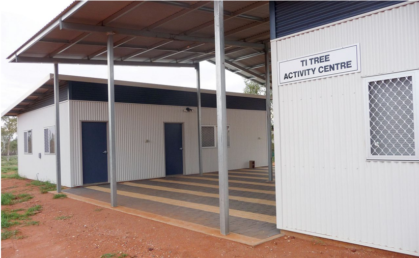
Fig. 6.9 New CDEP/RJCP Activity Centre and Office in Ti Tree 2013
