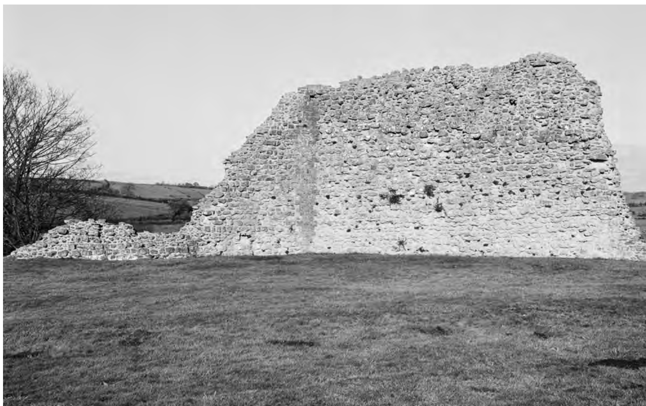
Fig 34 The remains of the curtain wall at the north-east corner seen from within the bailey, showing the Ham Hill ashlar quoining in the angle of the wall junction. Photograph: NMR EH/B925739
