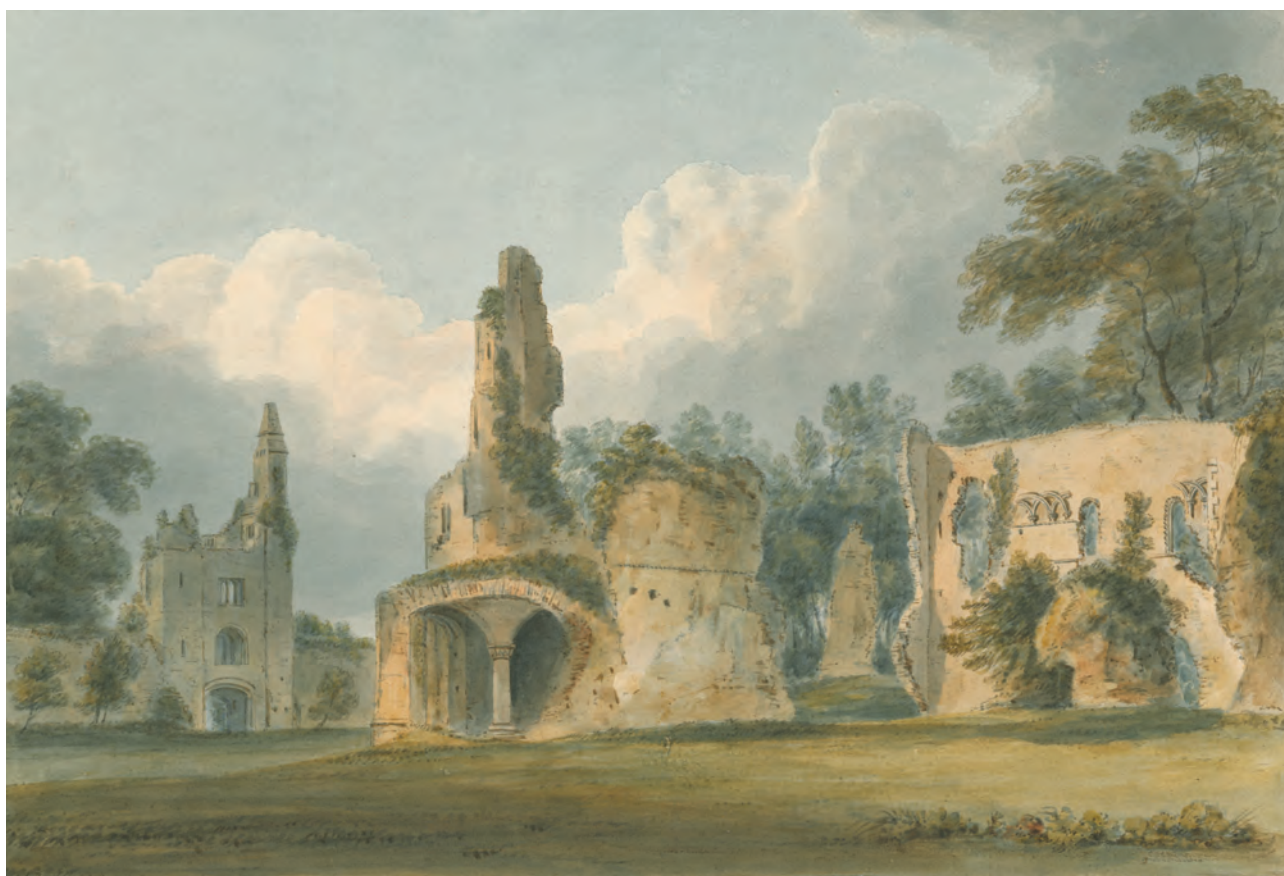
Fig 19 Watercolour view across the bailey from the east showing the remains of the central buildings and the south-west gatehouse tower to the left, by J Buckler, dated 1802. Photograph: William Salt Library, Stafford
