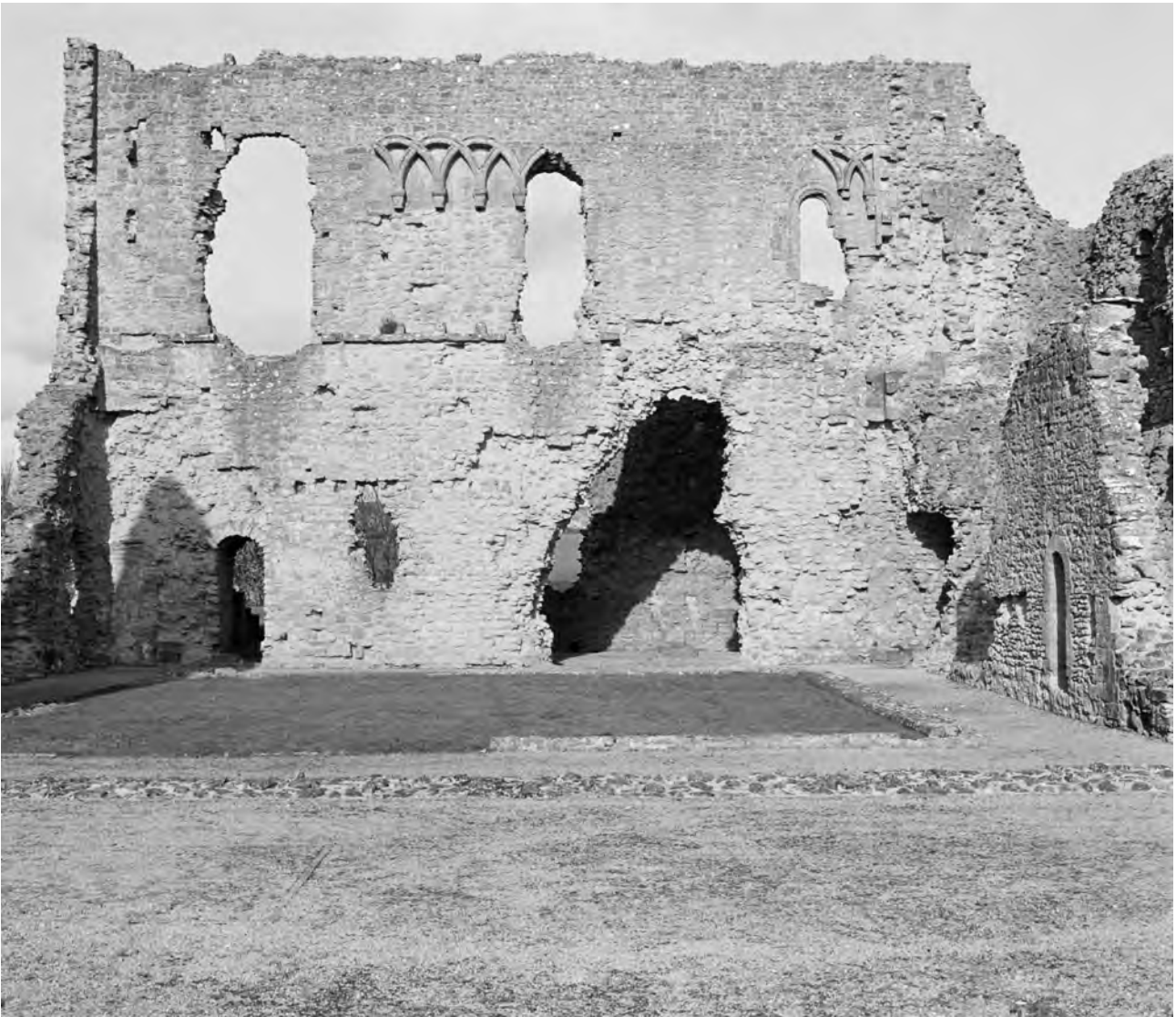
Fig 67 Central complex, north range: the south wall from the inner court. Photograph: NMR EH/B 925751
