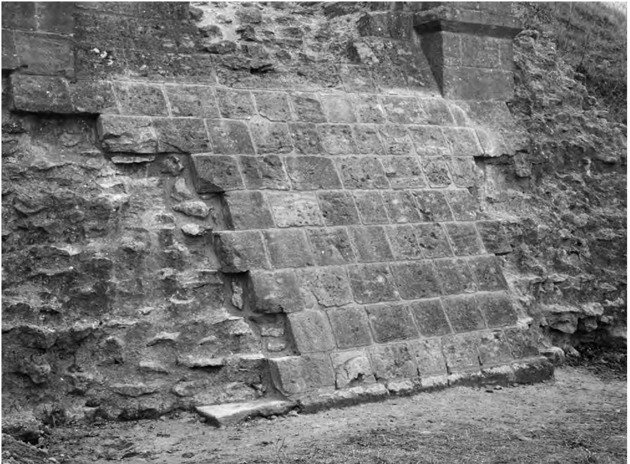
Fig 51 The north-east bridge: a detail of the ashlar-faced batter to the inner abutment of the bridge. Photograph: NMR EH/B905617
