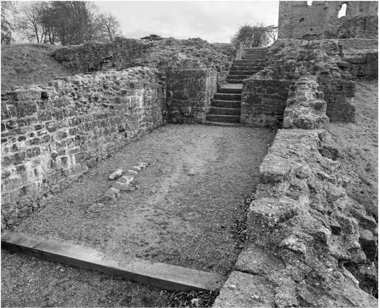
Fig 56 The north gate: the remains of the walled causeway leading to the stairs within the later gatehouse tower abutting to the curtain wall. Photograph: NMR EH/B925755
