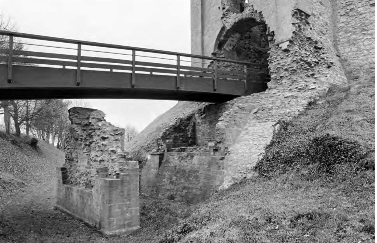
Fig 47 The south-west bridge: the central pier of the original bridge and the batter of the inner abutment, altered later to incorporate a drawbridge pit. Photograph: NMR EH/B925724
