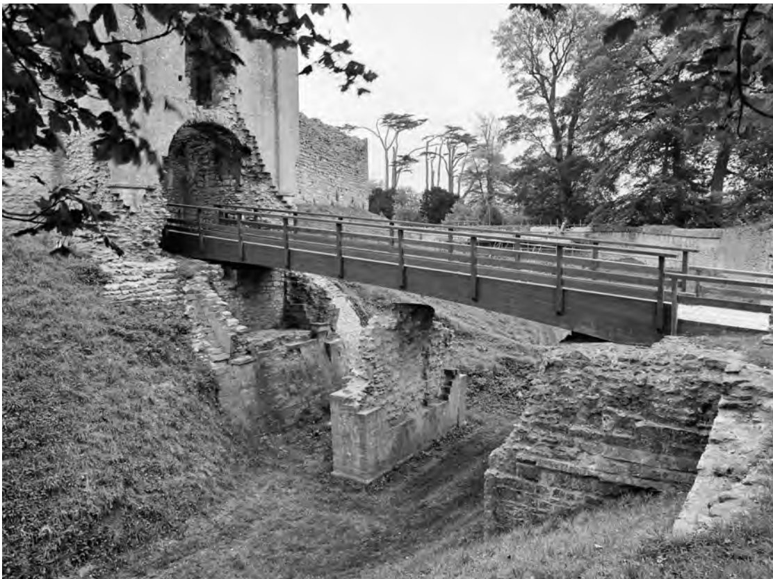
Fig 40 The south-west bridge: the remains of the twelfth-century bridge within the outer ditch seen from the west showing the central pier and the outer and inner abutments below the modern bridge. Photograph: NMR EH/B925719
