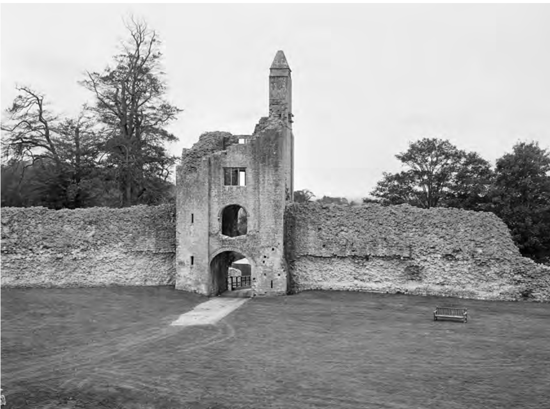
Fig 36 The south-west gatehouse tower and the flanking lengths of the curtain wall seen from inside the bailey. Photograph: NMR EH/B925711
