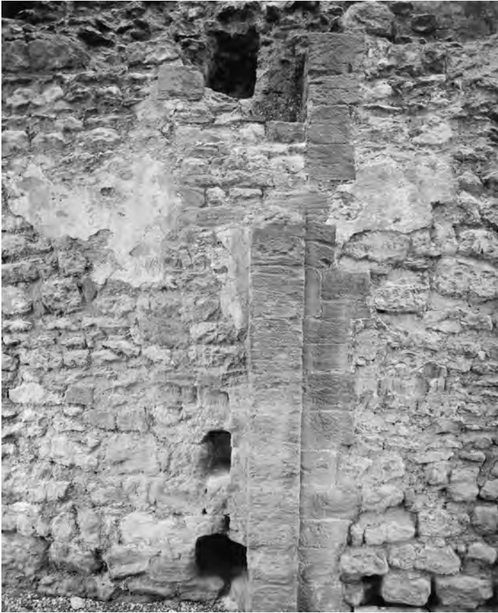
Fig 39 The south-west gatehouse tower: a detail of the ashlar jamb at the centre of the south-east side of the passageway through the tower. Photograph: NMR EH/925733
