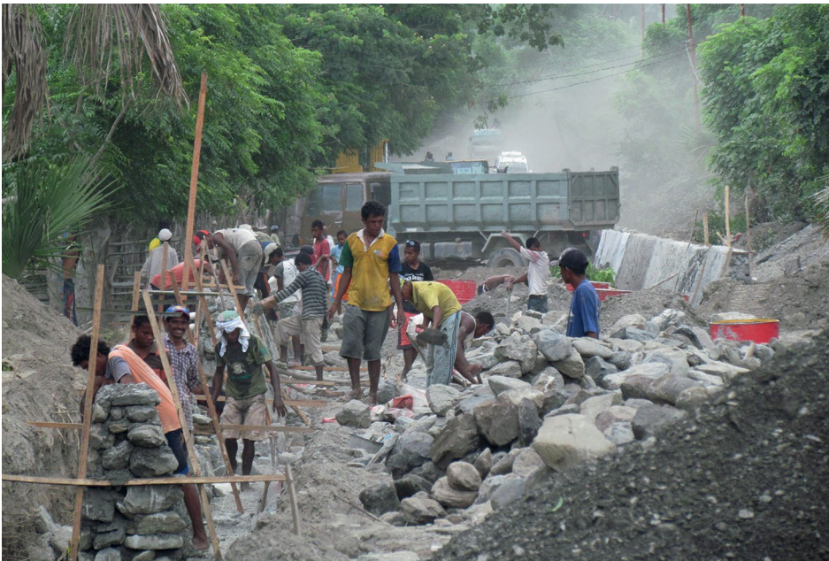
Figure 7.1 National road upgrading project.
