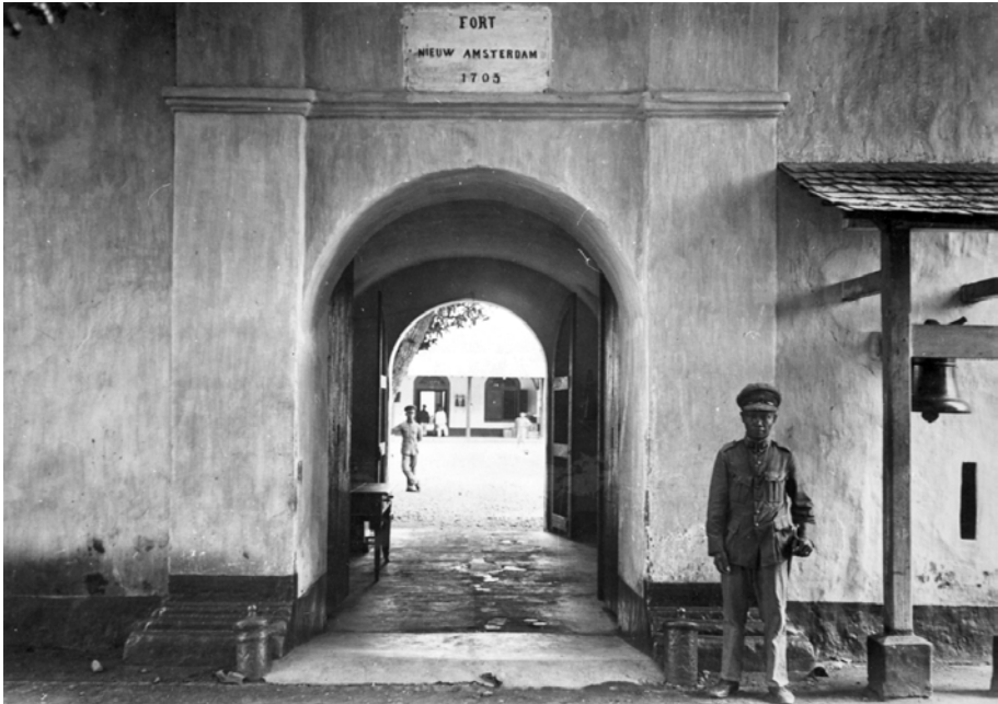
Plate 78. 'Fort Nieuw Amsterdam', Manado (completed in 1705) where Dipanagara was kept between June 1830 and June 1833. The Resident's house in which he had his accommodation can be seen through the open gateway. The fort was later destroyed by American bombing (circa 1944). Photograph probably taken in the 1930s. Courtesy of the KITLV, Leiden.
