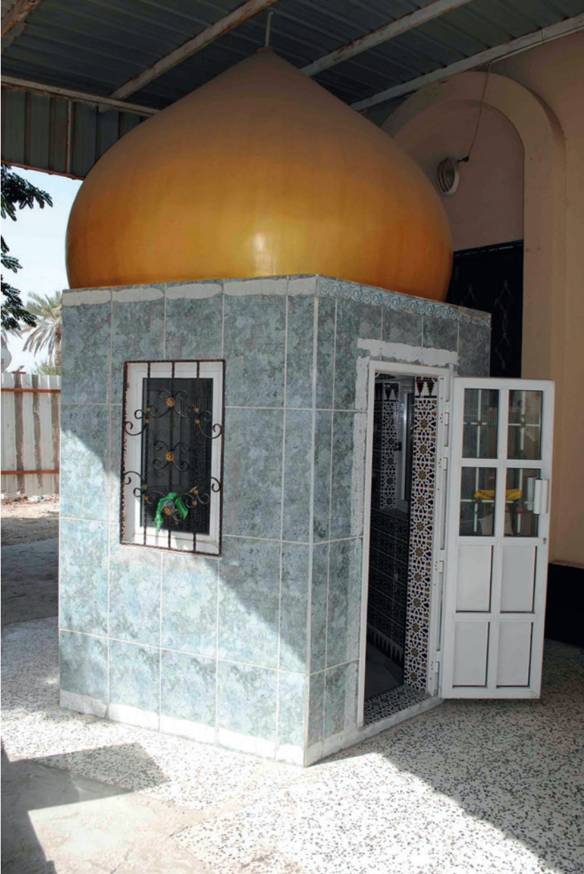
FIGURE 3.25 Domed shrine containing SYA1, Sayed Yahya Al Husseini mosque
