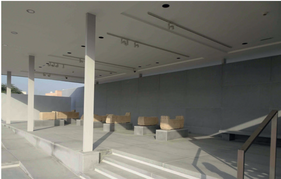
FIGURE 3.31 Gravestones raised on granite plinths in external pavilion, Al-Khamis Mosque visitors centre
