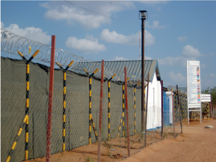
I.II. CARE compound gate and guardhouse, WFP sign listing international partners, on the main drive through humanitarian compound at Dadaab.
