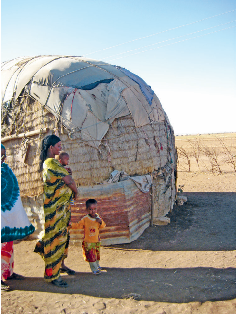
2.8. Tuqul clad with animal skins, harar (woven grass mats), and textiles, pictured here with the designer/builder and her children, Kebribeyah, Ethiopia, 2011.
