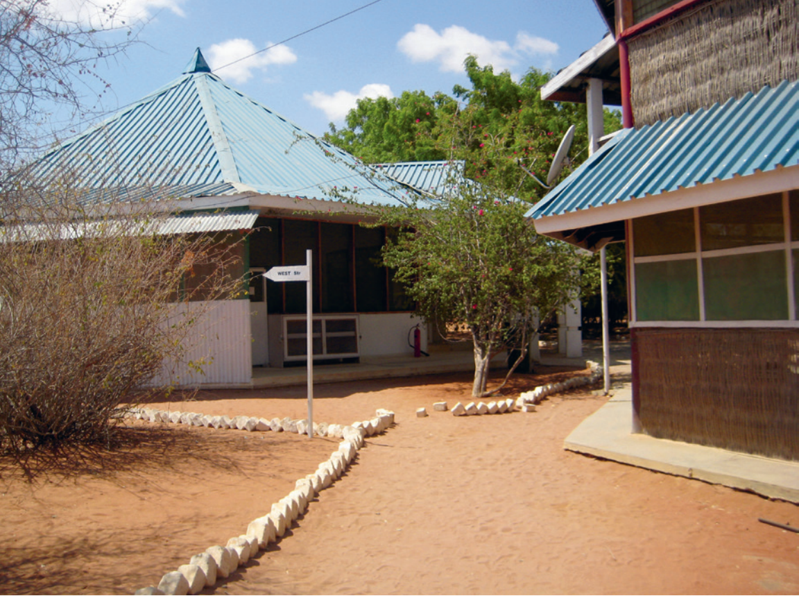
4.14. Mess hall and recreational center, UNHCR compound.
