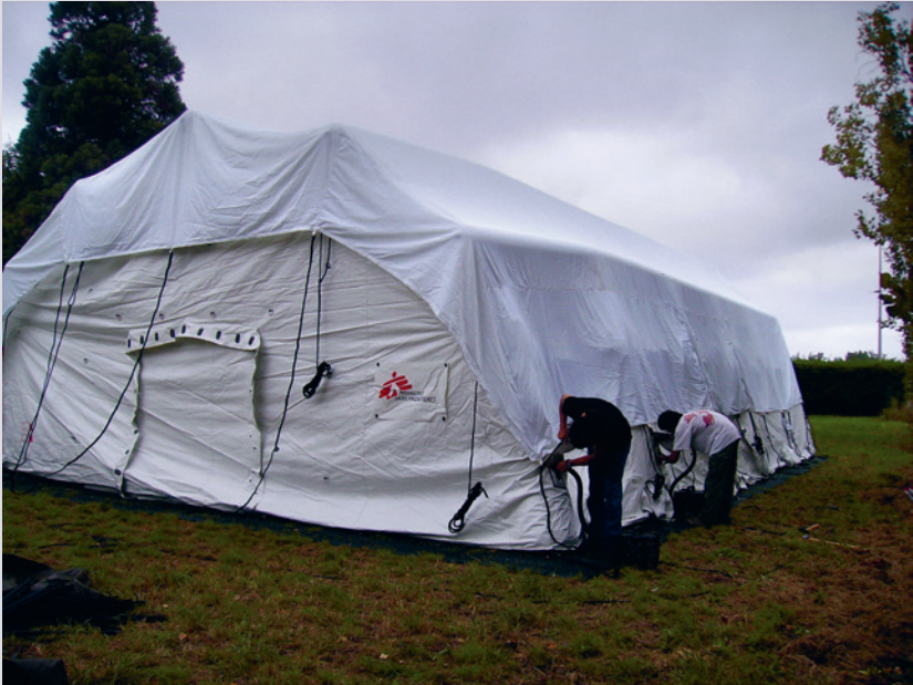
5.12. Inflatable hospital prototype, Mérignac, photo provided by MSF Logistique.
