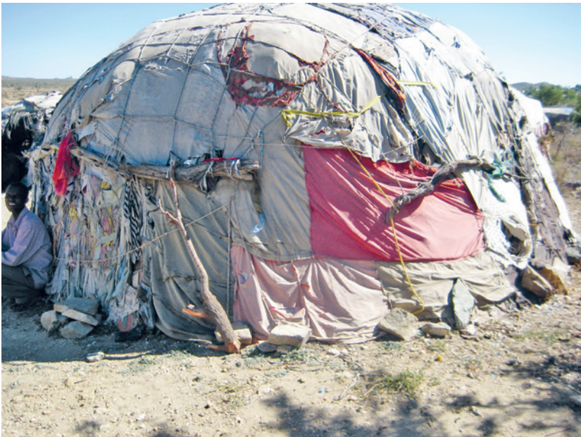
3.8. Tuqul constructed from recovered textiles (location undisclosed to retain privacy).
