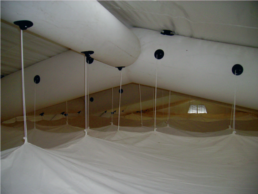
5.14. Inflatable hospital prototype, roof beam detail, Mérignac, photo provided by MSF Logistique.
