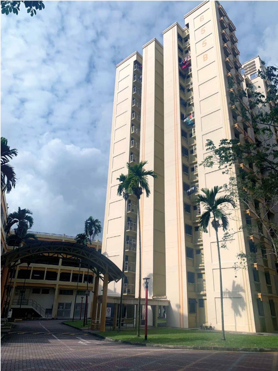
Figure 12.2. A typical HDB block in Jurong West, Singapore, with a signature block number on the building (photographed by the author, January 2020).
