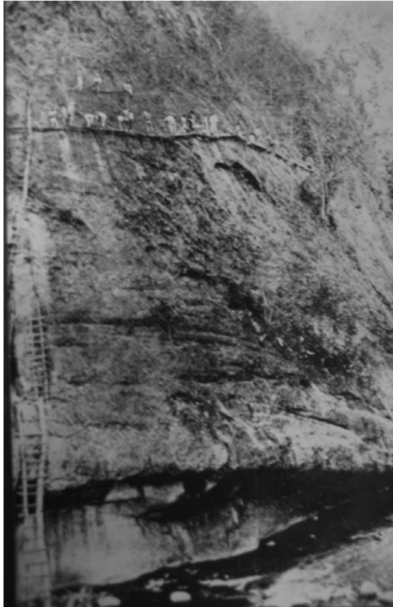
Figure 4.2 Road work in the Bued River Valley. In this unidentified surviving image of ledge work on the sheer mountainsides of the Bued River valley, we can make out the ladders extending upward from the lower left corner of the image to a high ledge or platform on which the figures of perhaps 20, likely conscripted workers can be seen chipping away at the side of the mountain under precarious conditions.
