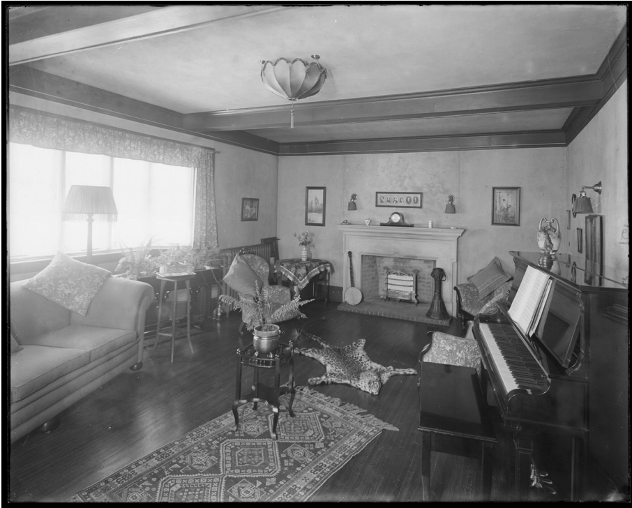
Figure 1: Living room with gas radiant fire, hot water radiator, gas and electric lighting, leopard skin rug and piano. F.W. Micklethwaite's Studio, 1913. City of Toronto Archives, Fonds 1034, Item 887. Public Domain.
