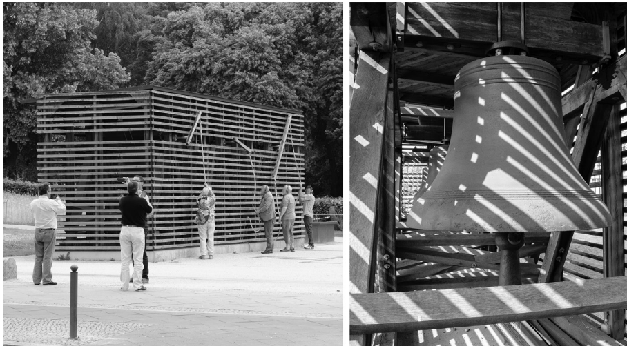
Figure 6: Photos of the contemporary wooden shelter in a gravel plaza, in which the original church bells are suspended. Image at left shows local volunteers ringing the bells before a memorial service held in the adjacent chapel; image at right shows the three bells. © the author.
