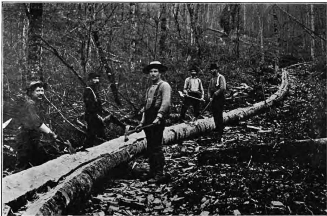
BUILDING A SLIDE. (CORBETT, PA.)
