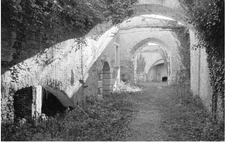
Fig. 1: Giorgio Andreotta Calò, Fort of Sant'Andrea, Venice, 2024, Walkways inside the bastion.
