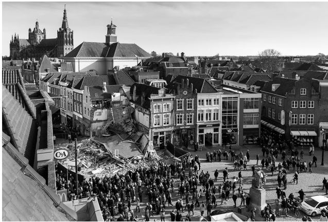
Photo 8.2 The collapsed building next door to the former house and studio of Bosch (photo: Marc Bolsius).
