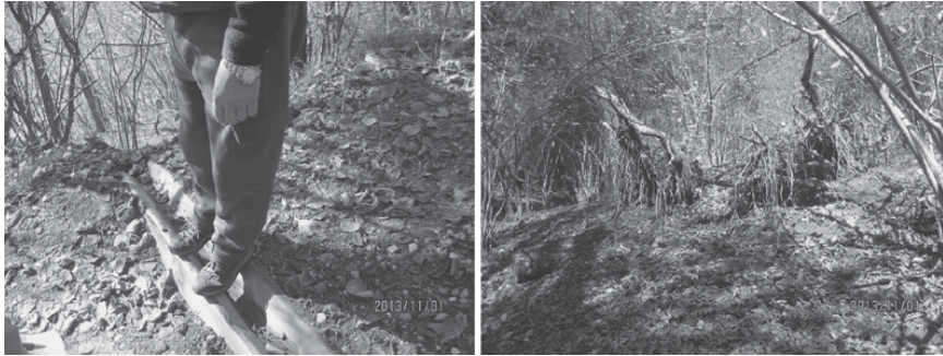
Figure 7.7 Nature walk, a blocked drain, uphill (left), and neglected woodland (right), November 1, 2013.
