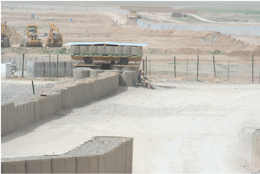
Figure 6.5: An example of a Hesco bastion in Camp Holland. 27
