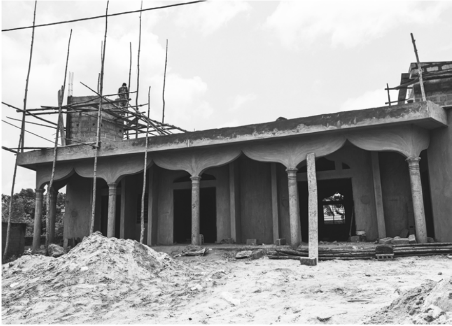
Fig. 15: ACEEMUB Mosque under construction, 16 March 2022, photo by the author.
