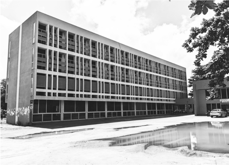
Fig. 12: ILACI building, 12 June 2024, photo by the author.
