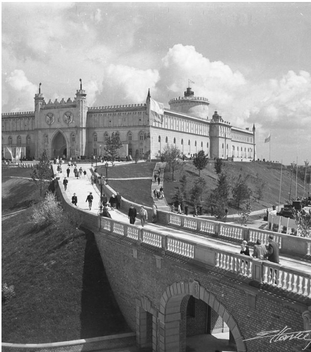
Figure 7.5 Lublin Castle Viaduct.
