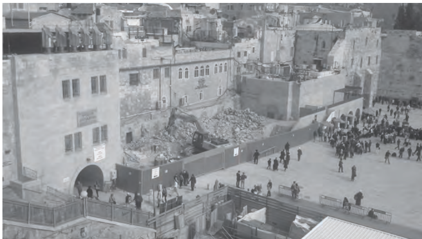
Figure 2.3 Demolition of part of the old building before the limited excavations. Photo Emek Shaveh
