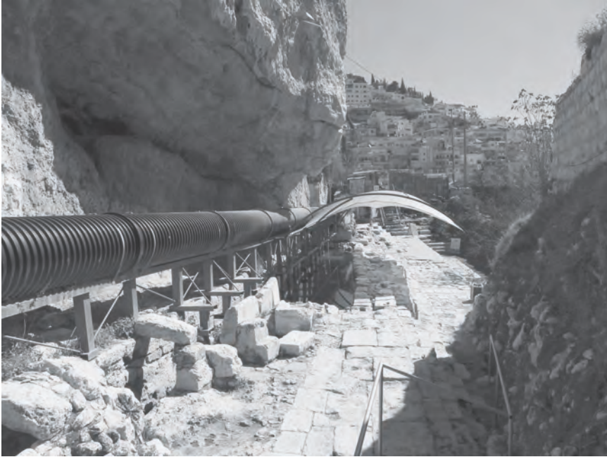
Figure 1.13 Sewage pipe at the Siloam Pool.
