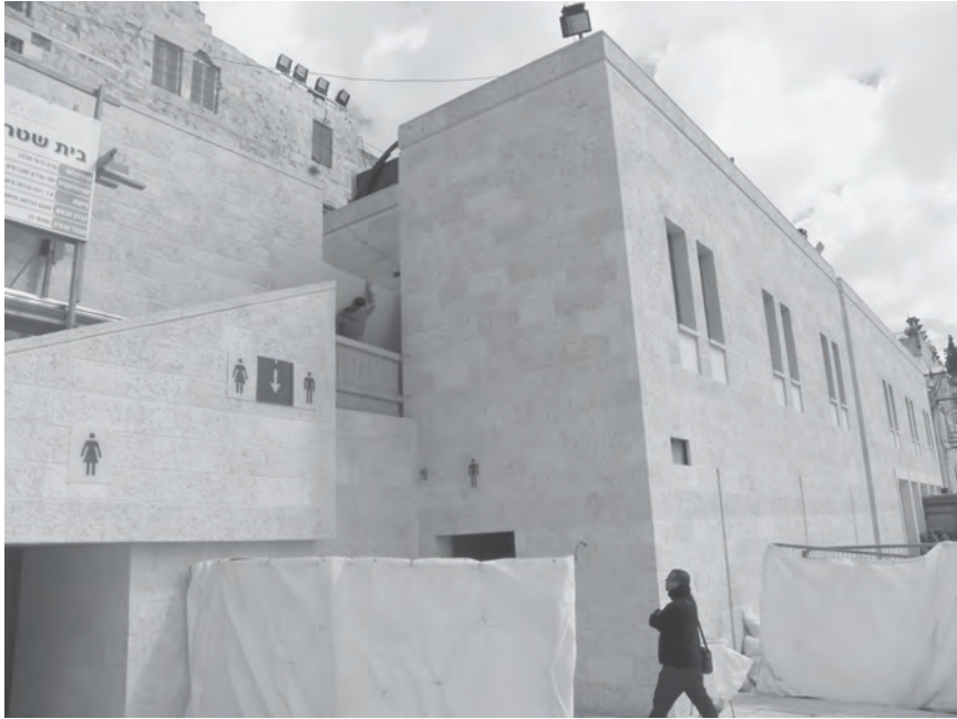
Figure 2.6 The Strauss Building after the extension (2015).
