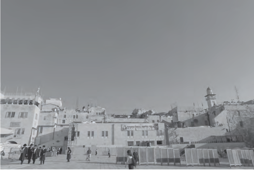
Figure 2.2 The Strauss Building after enlargement, view north from the Western Wall Plaza.
