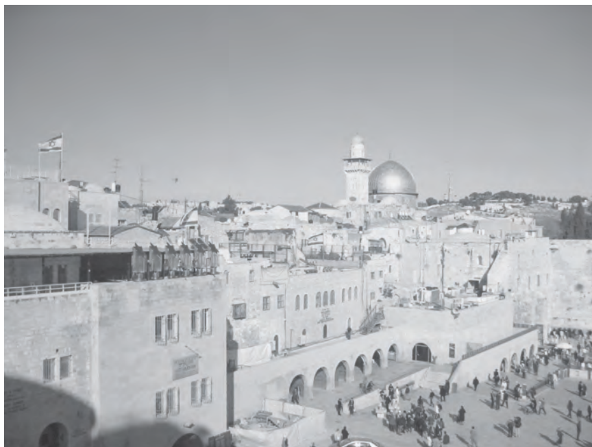
Figure 2.1 The Strauss Building (at centre) before the enlargement; the Western Wall on the right.
