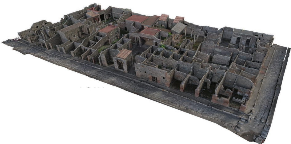
Figure 3.6 3D model of the insula V1, Pompeii. The Model was acquired by combining Laser scanning and image-based 3D Modelling techniques. Once created, the model was georeferenced and imported into the 3D GIS platform used during the investigation. Image courtesy of the Swedish Pompeii Project.
