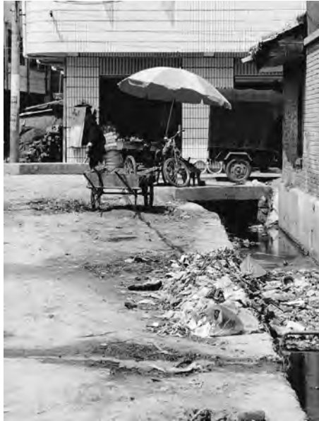
Photograph 5 Wulong township in Yunnan province.
