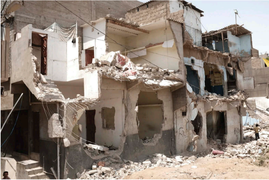
Figure 11.5 Houses demolished in Moosa Colony, located along the KCR track Source: KUL photo archives, 2019.
