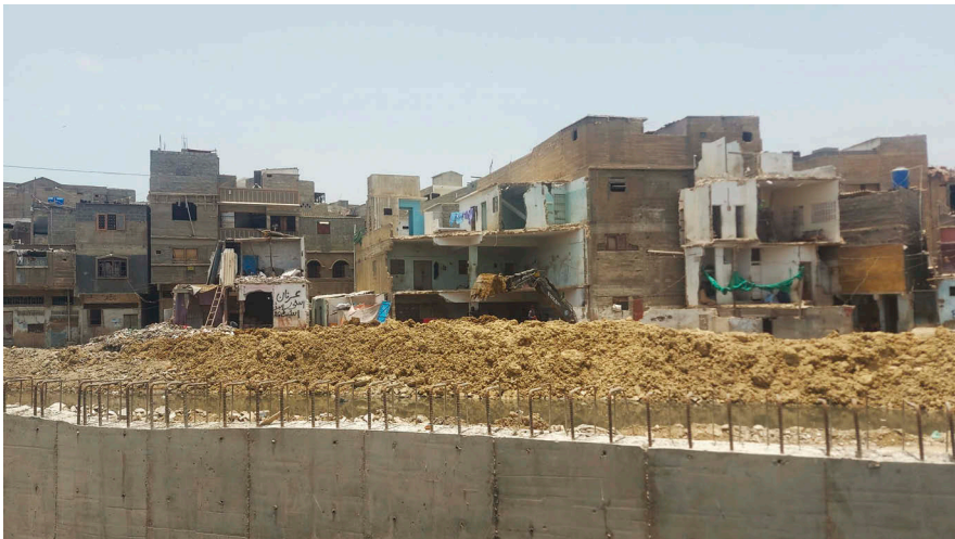
Figure 11.8 Demolitions in Kausar Niazi colony, a settlement located along the Gujjar Nullah, to make way for storm water drainage
