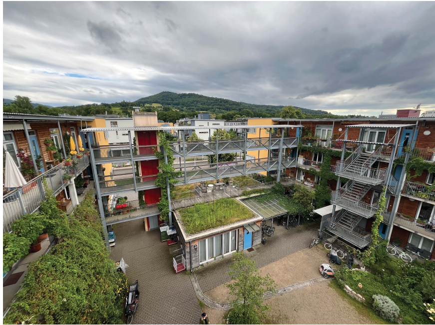
Figure 2.5.2 The Genova project in Vauban is a modern-day hous- ing cooperative with 72 units. Photo by author.
