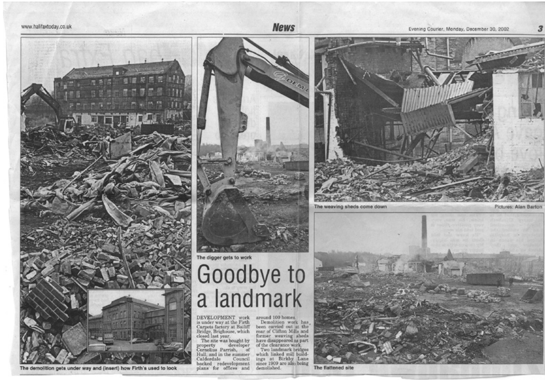
Figure 1.16 Local press report the demolition of Clifton Mill, 2002. Author's newspaper cutting.
