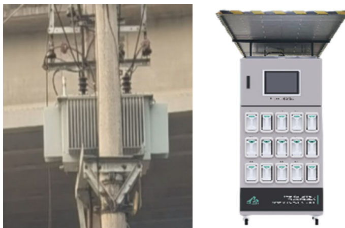
Fig. 7.12 Application scenario of integrated PV-storage-charging-swapping-testing cabinet in the transformer coverage area
