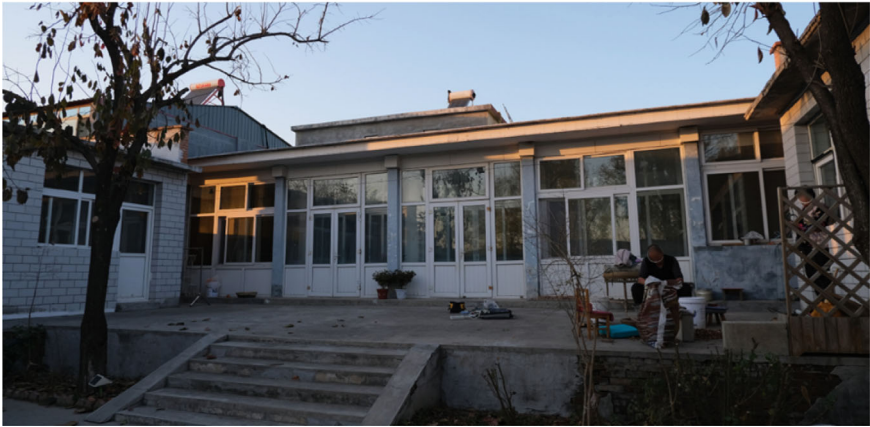
Fig. 3.19 Floor plan of RRB for comparison testing of heating equipment a Floor plan; b RRB photo
