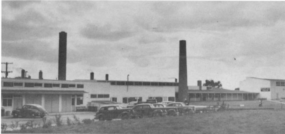
Willow Lodge Management Office and Post Office
