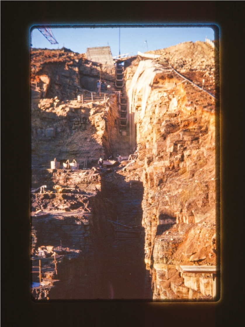
Figure 2.3 Cross-section of eastward dam with workers, 1960s, Washburn Heritage Centre
