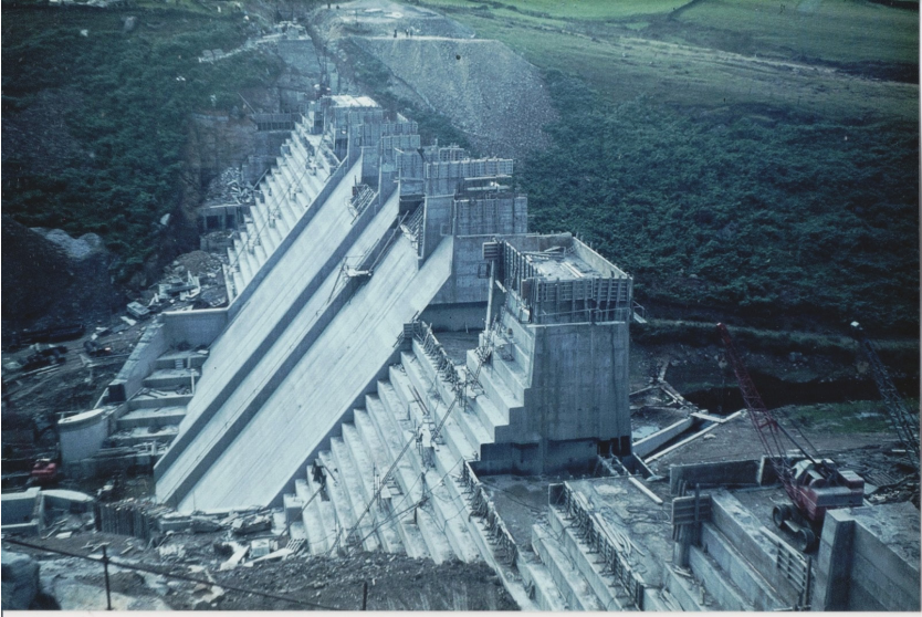
Figure 2.2 Thruscross dam during construction, 1960s, Washburn Heritage Centre
