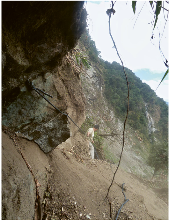
FIGURE 37: Destroyed road near Panang HEP site, November 2011.
