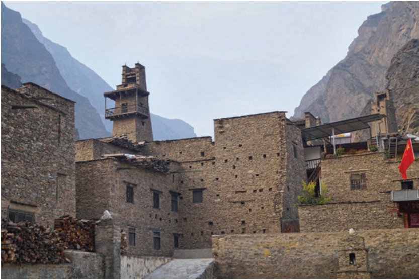
Figure 5. Overview of Taoping Qiang Village. Photograph courtesy of Jingui Zhang.
