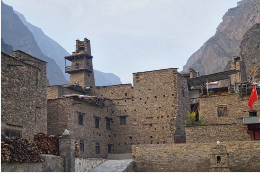
Figure 15. Overview of Taoping Qiang Village. Photograph courtesy of Jingui Zhang.
