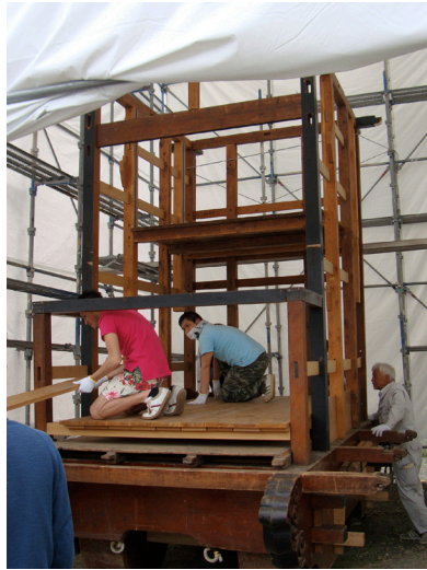
Figure 6 The Nishimachi float of Chiryū as it is being assembled. The last board of the bottom level is put in place by the man kneeling in the front part of the float. The upper level can be seen above the man kneeling in the back. There is no middle level in this float, but at the bottom it has the remainder of a no longer used stage floor, which could be pulled out forwards for puppet performances (29 April 2017).
