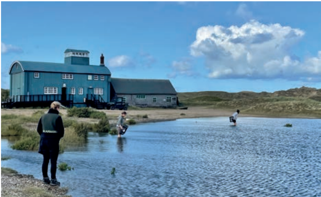
Students and researchers at the UCL Francis Wall Oliver Field Station. The low grey building in the background is the original lifeboat house on Blakeney Point, and dates from the nineteenth century. The blue building is the new lifeboat station, which now houses National Trust wardens and exhibits.
