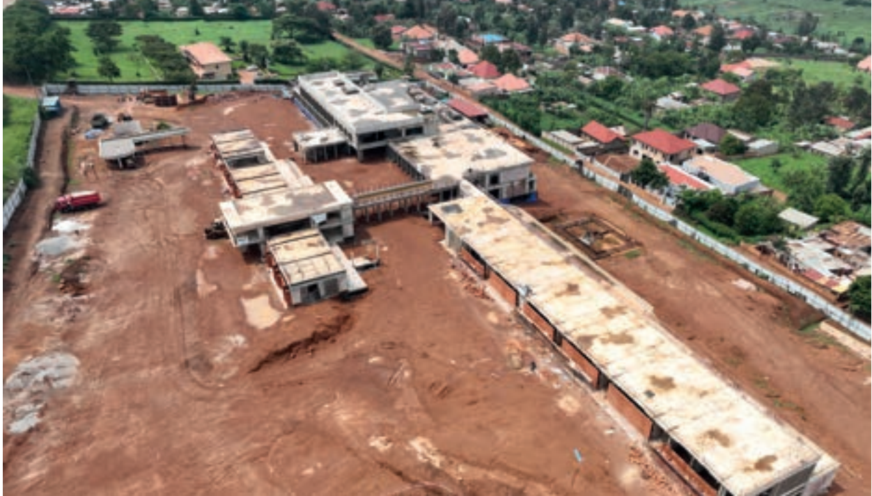
Construction site in Rwanda, November 2024.
