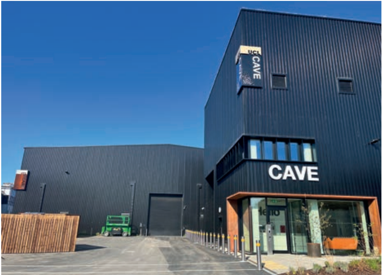
The CAVE facility, opened in 2023.
