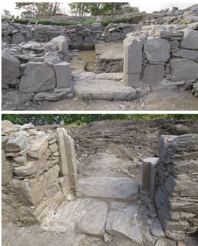
Fig. 6.22: The 1.28 meter wide cellar doorway oriented towards the harbour in the east is one argument for interpreting the cellar as a storage room. Pictures showing the doorway seen from the outside (facing west) and inside (facing east). Both doorjambs have inward facing rebates, meaning the door swung inwards. Photo: MCH.
