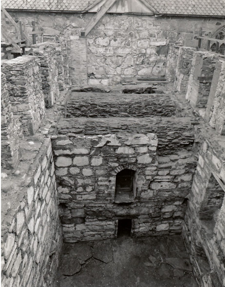
Fig. 7.23: Utstein. The possible royal residence at Utstein, viewed from the south. Visible are the southernmost cellar and basement, and the barrel vault over the two other rooms. The walls of the first floor are post-medieval. In the background are visible parts of the abbey church. Photo: G. Fischer. Source: The Directorate for Cultural Heritage.
