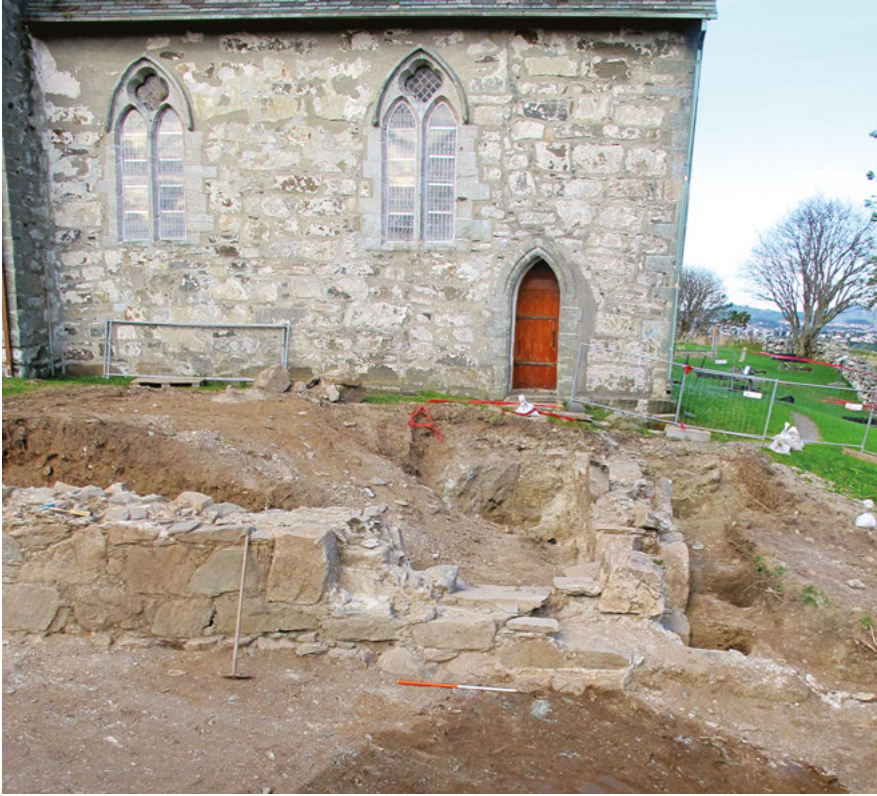
Fig. 6.16: High-quality masonry, A60010 (forefront) and St Óláfr's Church chancel in the background (compare Fig. 6.11). Above the western side of the chancel portal there appears to be an unbound vertical joint of several meters (facing north). Photo: MCH.
