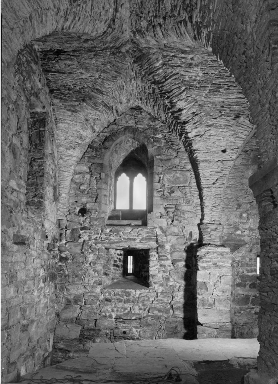
Fig. 7.7: The royal palatium at Holmen. King Håkon's hall, the two lower stores during restoration in the 1950s. The vaults, built after the fire in 1266, are constructed with thin flagstone. Photo: G. Fischer. Source: The Directorate for Cultural Heritage.
