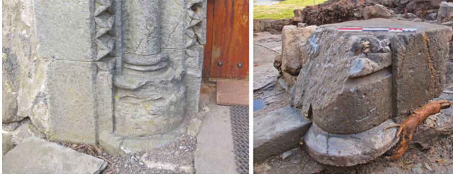
Fig. 6.13: The southern nave portal of St Óláfr's church to the left, and the southern column base of A60010's western portal to the right. Both with the same dog-tooth ornament, although damaged in the latter case. Photo: MCH.
