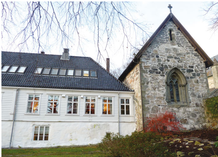
Fig. 7.33: Stavanger. The bishop's palace. The wing's basement in stone (now plastered) related to the two-stored bishop's chapel with the chapel itself in the first floor, viewed from the east. Photo: A. T. Hommedal.
