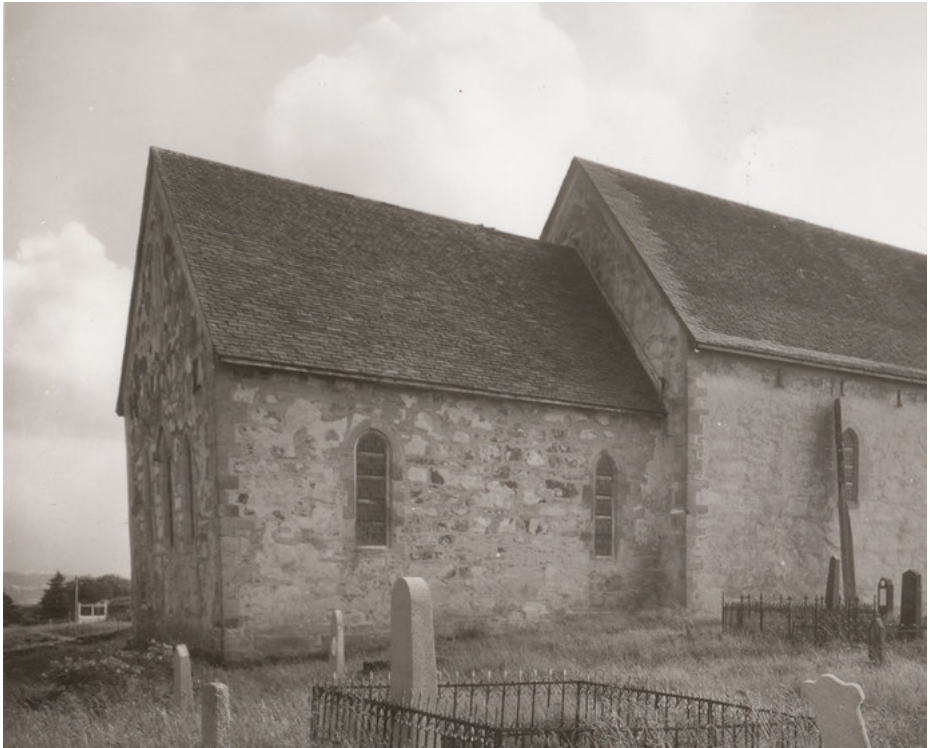
Fig. 6.18: The northern chancel wall of St Óláfr's Church, photographed in the 1930's. More recent photos obviously exist, but are seldom as clear. While the masonry is somewhat obscured by render, there are no obvious breaks in the north wall. The eastern side of the eastern window opening is much nearer the corner of the chancel on the inside than on the outside, due to the c. 1.5 meter thick walls and the much wider inside opening. In other words, the window could hardly have been placed further east. Originally published by: Norman. Photo: unknown, The Norwegian Directorate for Cultural Heritage's archives.
