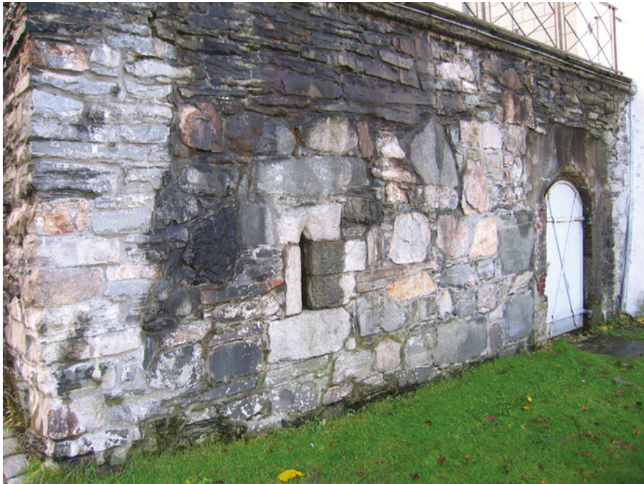
Fig. 7.28: The archbishop's residence in Bergen. A part of the early 14th-century masonry with its original small pointed window. Photo: A. T. Hommedal.
