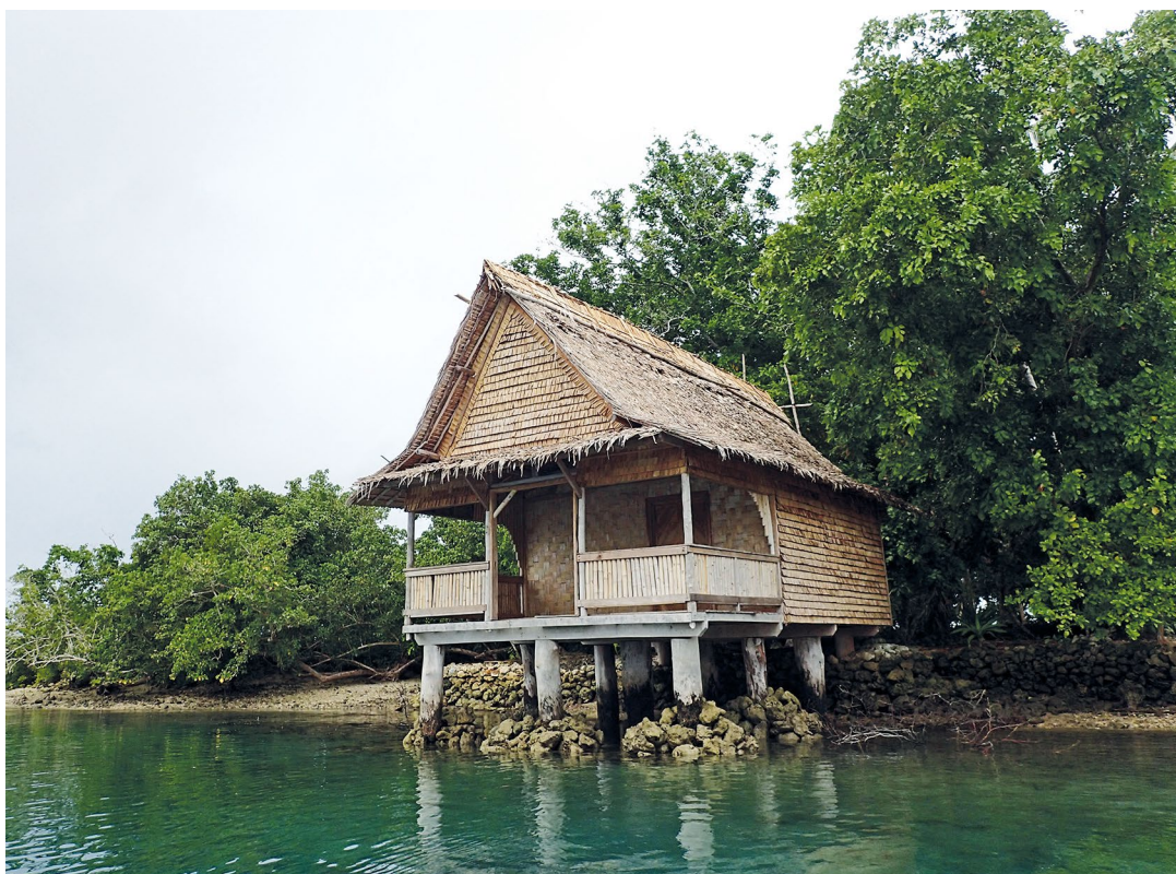
Figure 4.7. Dwelling in Langalanga Lagoon, Malaita, Solomon Islands, with limestone and coral boulders bracing sunken piles.
