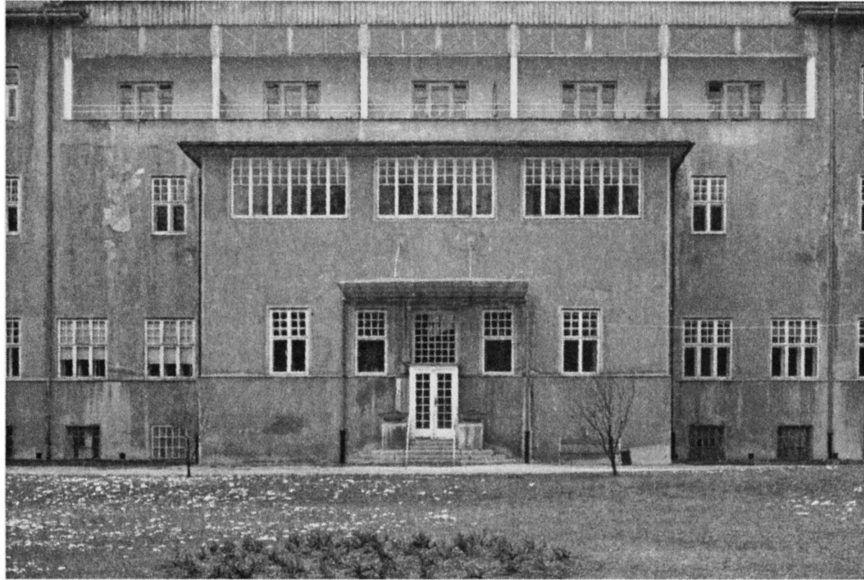
Figure 13. Sanatorium Purkersdorf, East Elevation (prior to restoration undertaken in the 1990s). Courtesy of Dario Galimberti.
