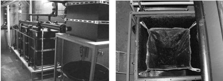
Figure 18.2. Vermicomposting batch reactors at the Hamburg University of Technology. Left: three batch reactors are connected to conventional flush toilets for the collection of faecal solids. Right: Interior of one reactor showing the filter bag during the collection phase (photos by courtesy of M. Shalabi).
