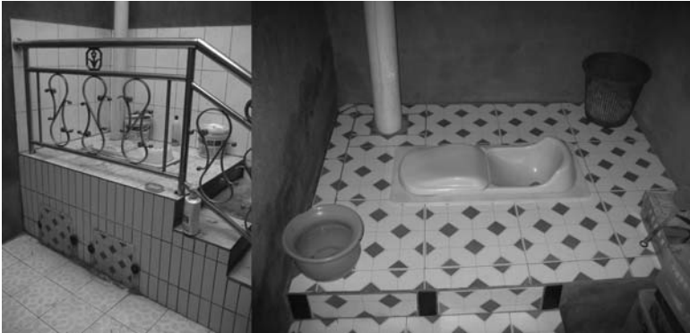
Figure 33.2 Typical (high-cost) situation of an in-house UDD toilet in the PLAN Shaanxi programme. A total of more than 2 million UDDTs were built in China between 2000 and 2010 (NDRC 2007). © Ph. Feiereisen
