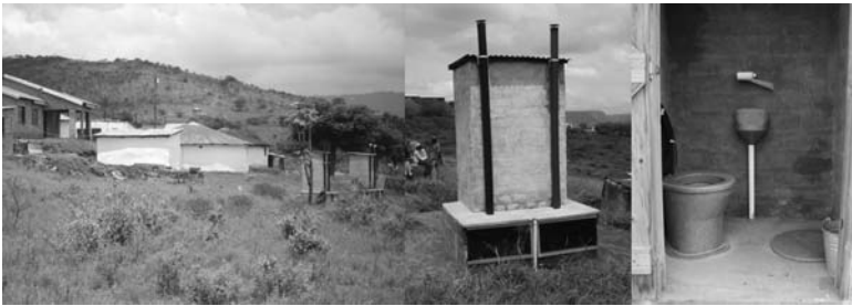
Figure 33.1 Images from left to right: peri-urban settlement with two UDD toilets on the right; a typical double-vault urine diversion dry toilet; inside view. © Duncan Mara
