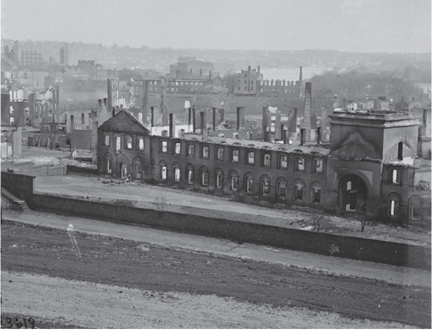
FIG. 1. April 1865 photograph by Andrew J. Russell shows the destruction of the waterfront across the canal basin in Richmond with the Virginia State Capitol and the U.S. Custom House in the distance. ( Library of Congress Prints and Photographs Division )
