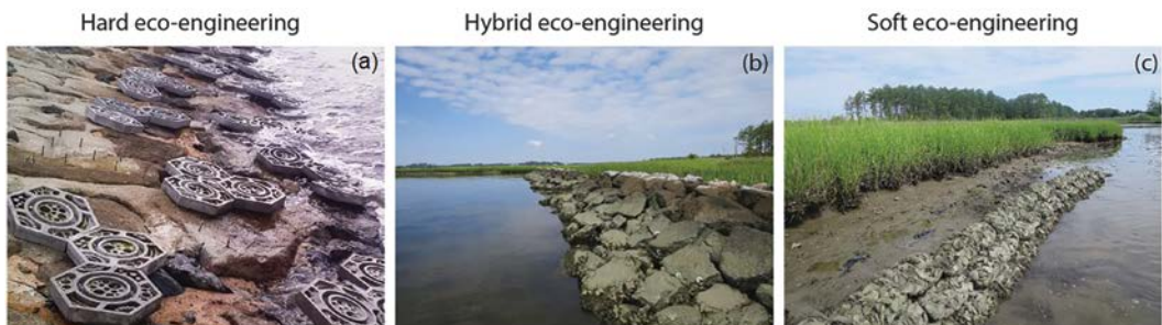
Figure 2 Approaches to ecoengineered shorelines include (a) hard (tile-enhancement units installed along the seawalls at Changi, Singapore), (b) hybrid (rock fillet with saltmarsh in Chesapeake Bay, United States) and (c) soft ecological engineering (bagged oyster shell reef with saltmarsh in Chesapeake Bay).
