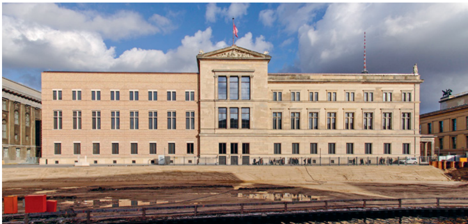
Abb. 7: Berlin, Neues Museum, Friedrich August Stüler, 1843–1855, Fassade zur Spree.
