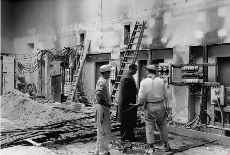
Fig. 4.10. Refitting the "Machine Hall," circa 1955.
