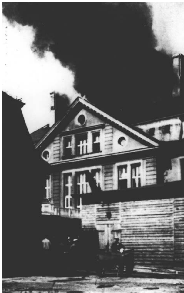
Fig. 2.13. Fire in the main building, 3 June 1925.
