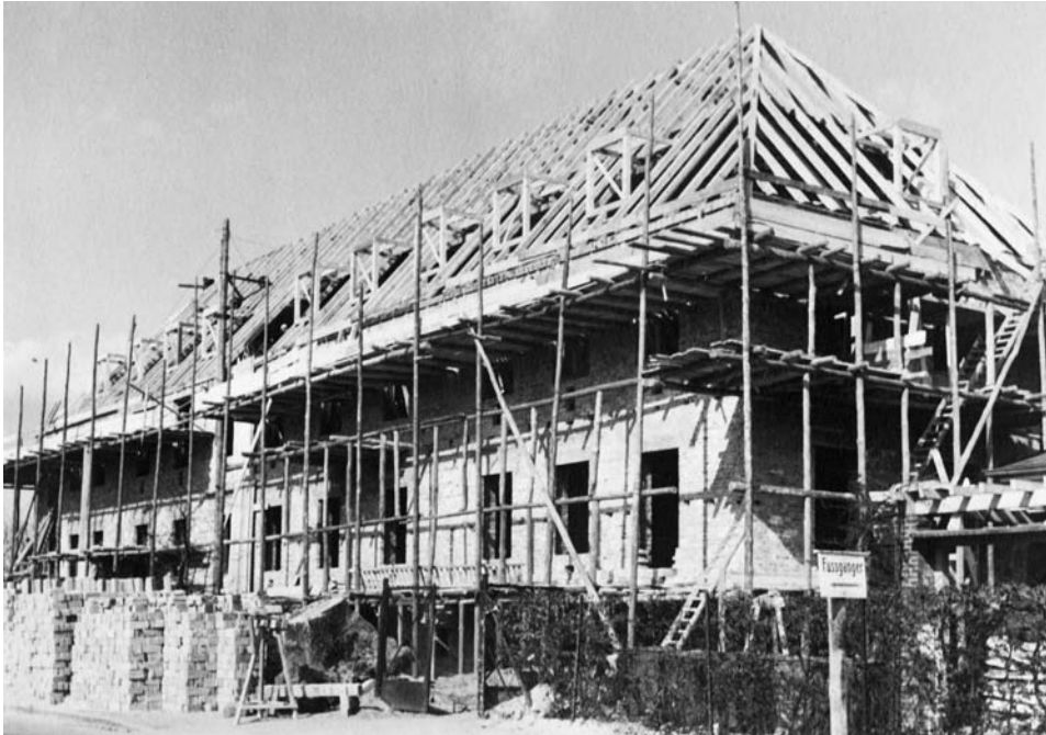
Fig. 3.12. Framing of the new X-ray building, 1938.
