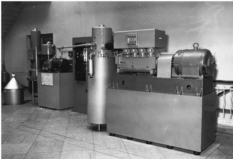
Fig. 4.11. The FHI helium liquefaction plant in the machine hall, 1958.
