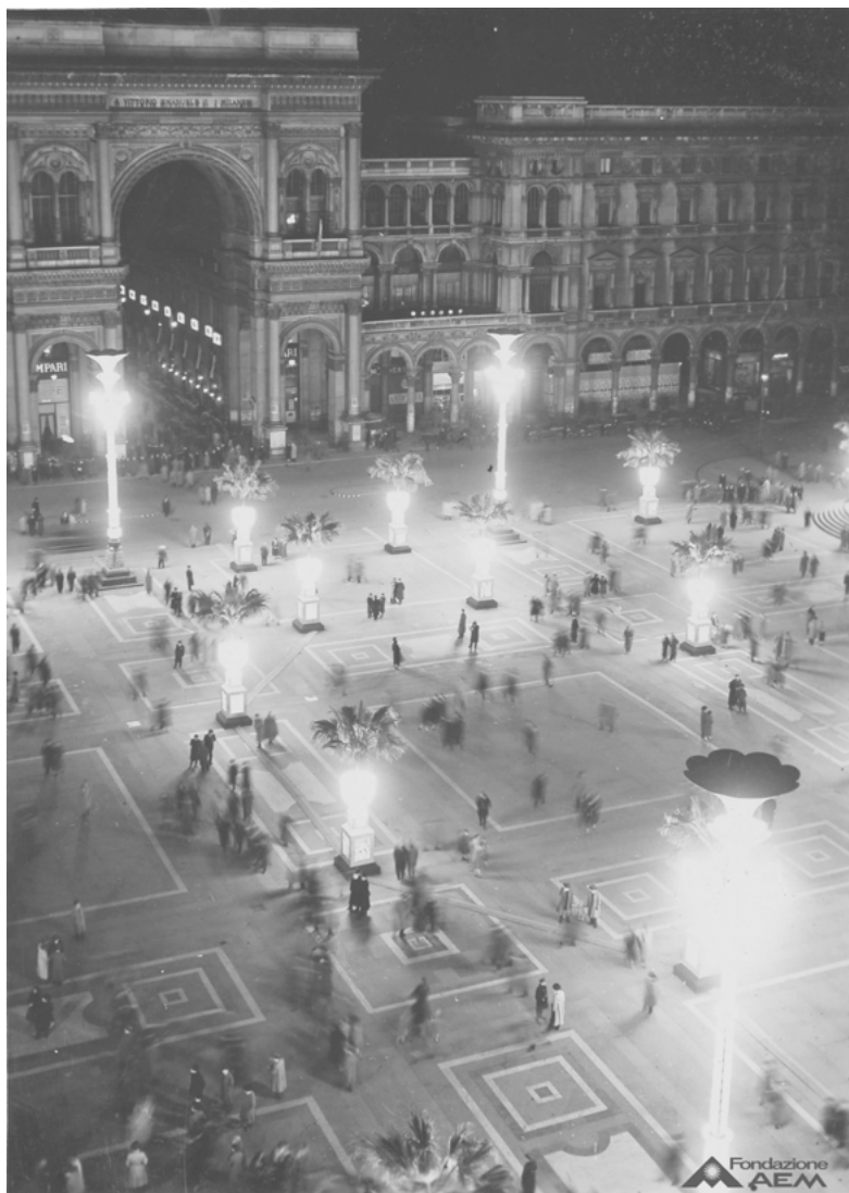
Figure 6: Installation of the illumination on the occasion of the anniversary of the March on Rome, October 28 th , 1933
