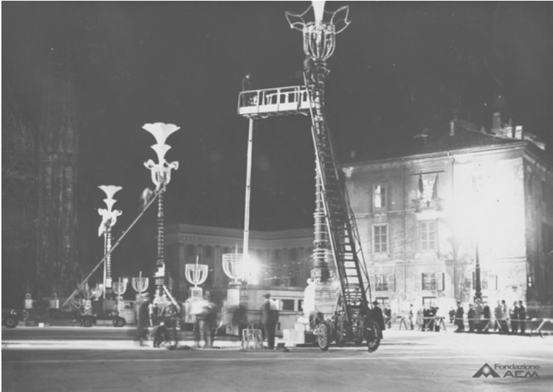
Figure 5: Installation of the illumination on the occasion of the anniversary of the March on Rome, October 28 th , 1933
