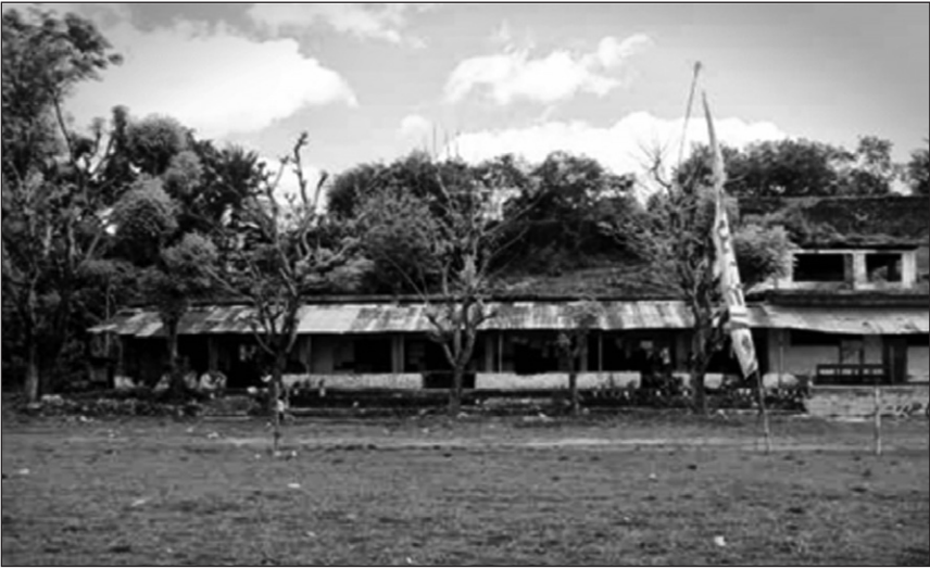
Merdeka Stadium (Freedom Stadium), Kupang City. Female detention centre.
