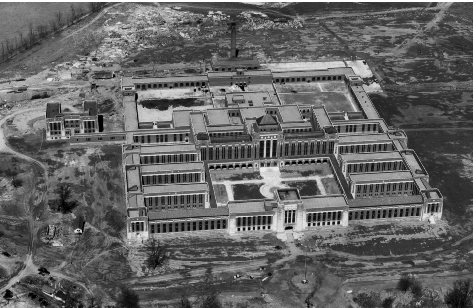
Aerial view of the institution at Lexington (1935). (Courtesy of the National Archives.)
