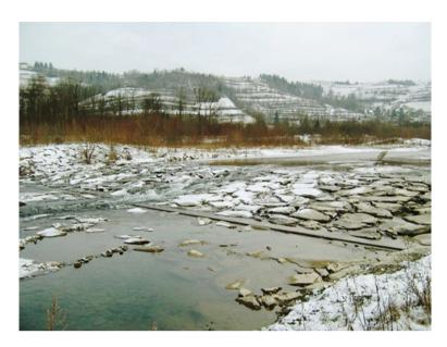
Fig. 5.9 Ramp—close to nature structure used in mountain rivers
