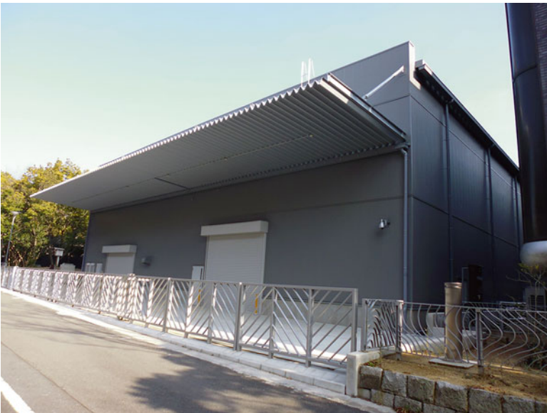
Fig. 6 Multi-functional storage facility storing wooden boats (after 2013)
