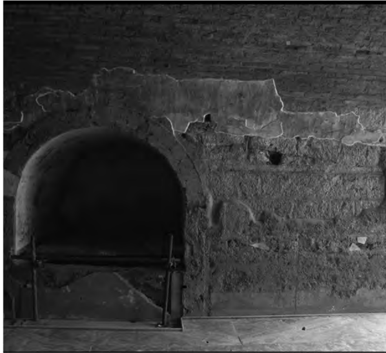
Abb. 6: Raum 36a, N-Mauer
