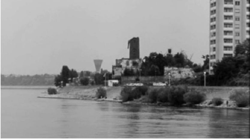
9 Vukovar, Croatia, with the water tower in the background.
