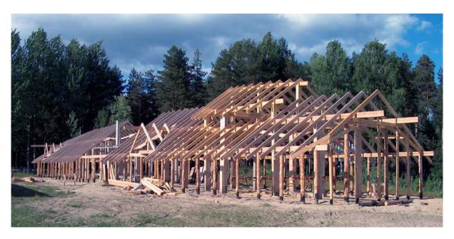
Figure 2. Photograph taken in 2003 during reconstruction of the large hall at Veien, Ringerike, Buskerud. Photo T. Bjørnstad, CC-BY-SA.
