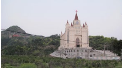
Sanjiang Church, Wenzhou, before demolition Source: Tom Phillips, Twitter
