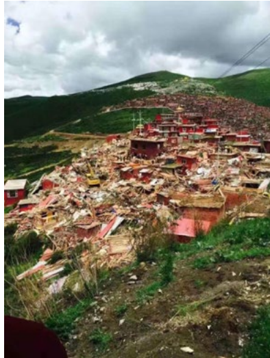
July 2016: The demolition of Larung Gar Source: Free Tibet, Flickr
