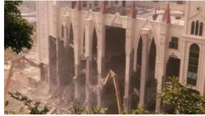
The demolition of Sanjiang Church Source: Guo Baosheng, Twitter
