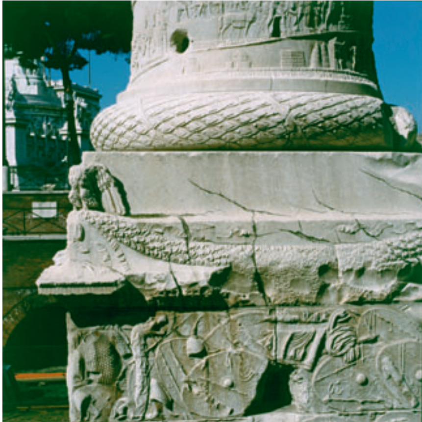
Fig. 5: The cornice of the podium, and the base of the column
