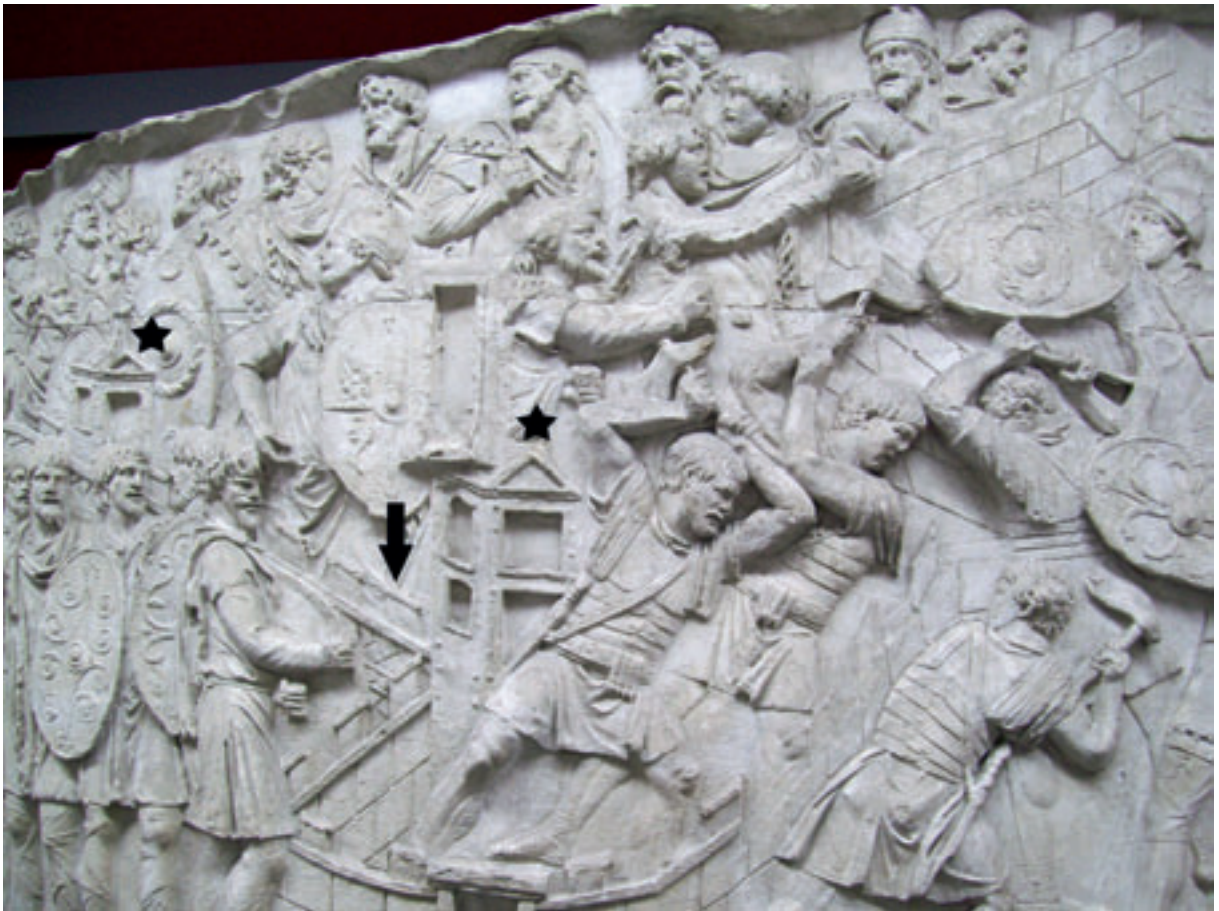
Fig. 12: Scene CXVI, Dacian fortifications. Arrow marks appearance of ashlar exterior for previously un-faced murus Dacicus ; stars mark tower buildings
